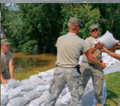
Indiana National Guard Soldiers pile sandbags on a levee in Hazleton, Indiana, to prevent a river from flooding nearby towns.
